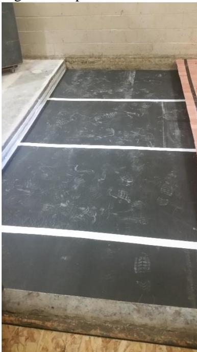
Figure 2 – Underlayment installed over concrete slab
