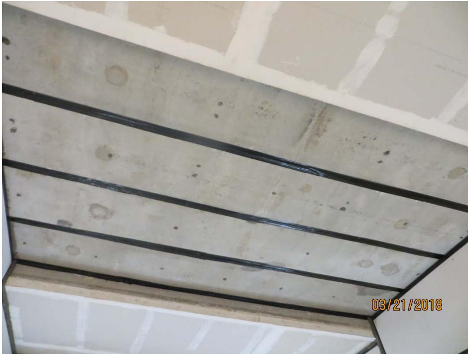
Figure 3 – Underside of test specimen
