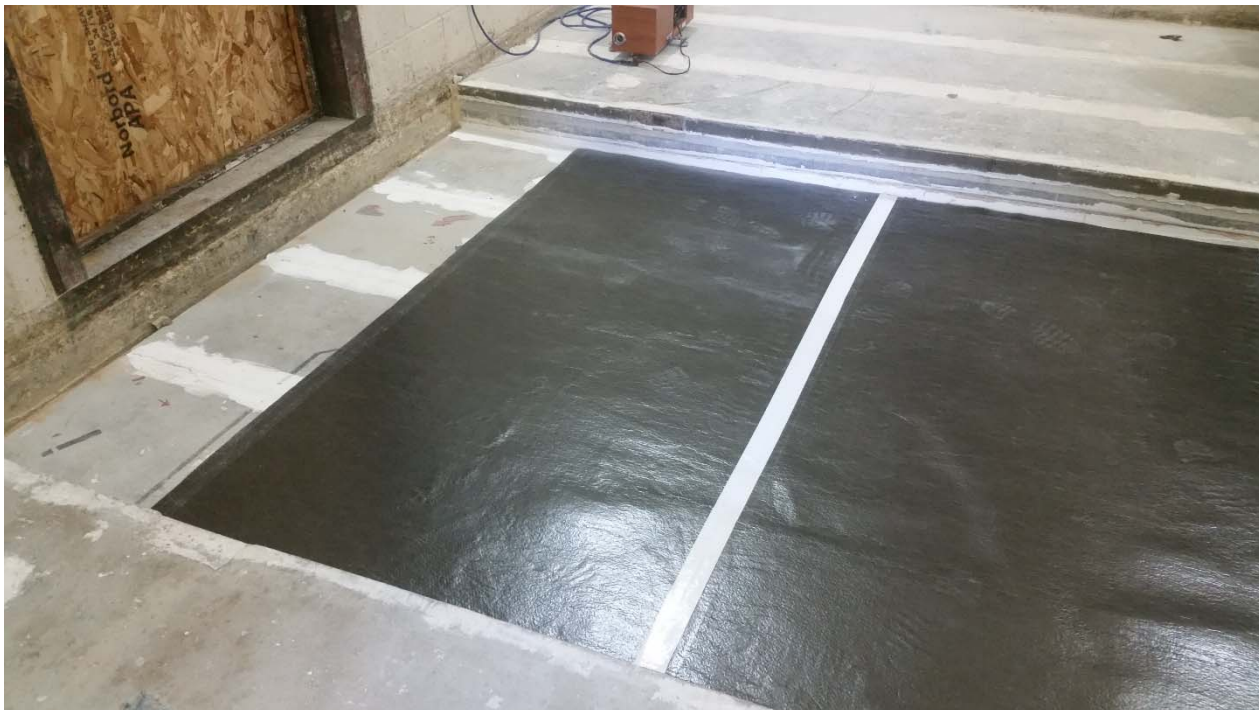
Figure 2 – Underlayment partially installed on concrete slab
